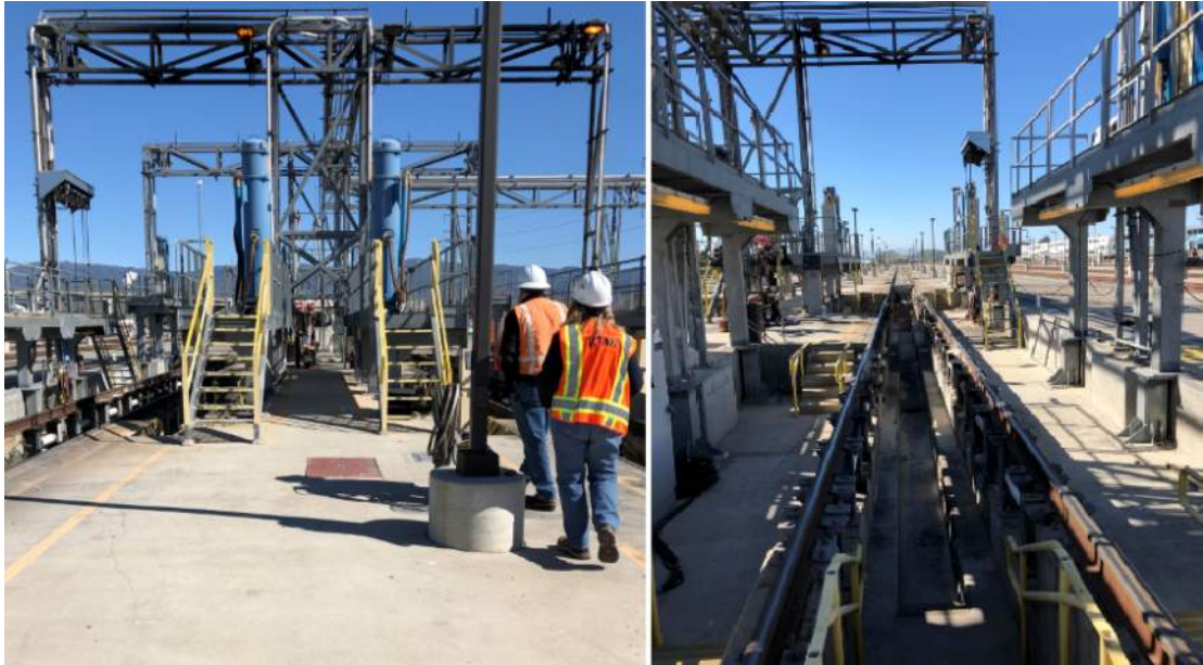
FIGURE 1-G. PLATFORMS AT END OF S&I POSITION
