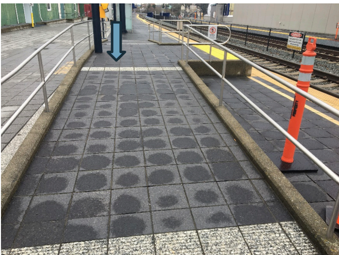
FIGURE 23: EXAMPLE OF MINI-HIGH RAMP
