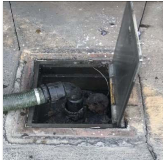
Ex. 17 – Proper Elbow Connection
