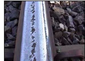
Severe Rail Center Spalling
