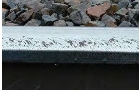
Severe Checking with Spalling
