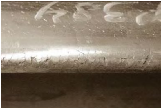
Head Checking with Flaking
