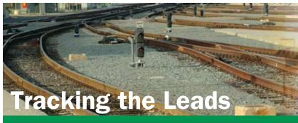
If you are one of the many Metrolink passengers that commute to Los Angeles Union Station, you may have noticed construction activity near the tracks as you approach the passenger loading and unloading platforms. This construction will improve the "leads," which are the tracks just past the turn from the Los Angeles River, allowing more trains to enter and leave the station in a shorter time.
