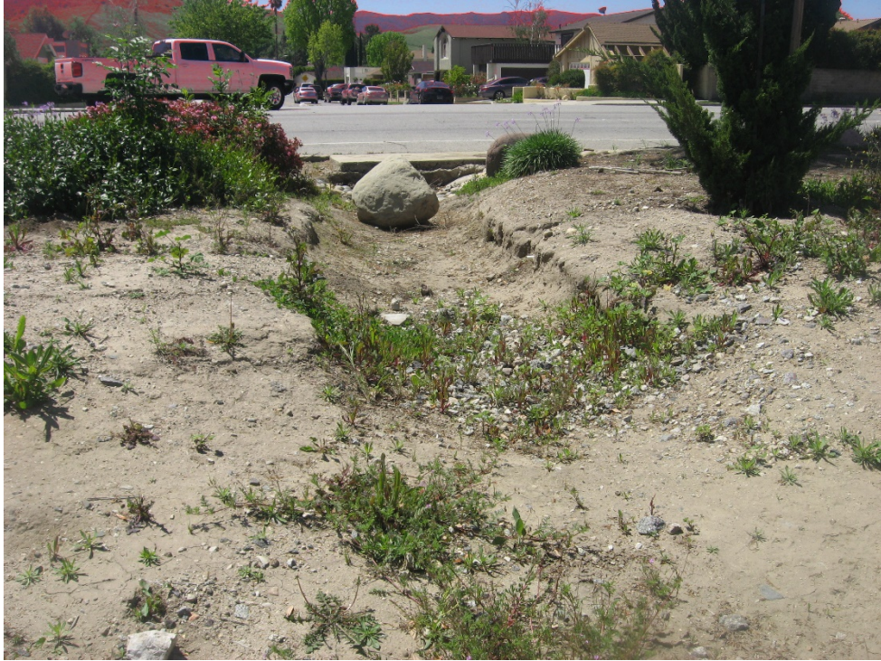
Photograph 11: Swale leading from culvert MP 436.56 to storm drain inlet at Los Angeles Ave. No OHWM. Slight historic incision visible for approximately 5 feet (4/21/2020).
