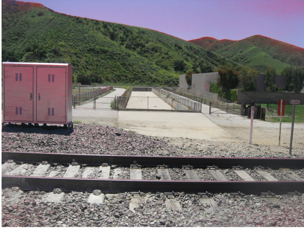
Photograph 17: Rail Right-of-Way looking south at Las Llajas Canyon channel (4/21/2020).
