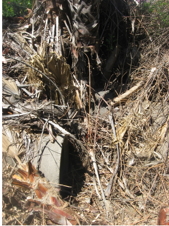
Photograph 5: 24-inch Culvert passing beneath the rail. No OHWM, bed or bank present (4/21/2020).
