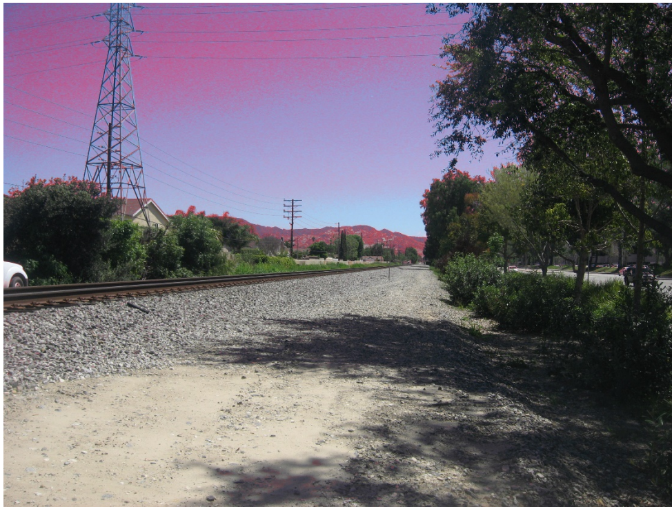
Photograph 16: Rail Right-of-Way looking east (4/21/2020).
