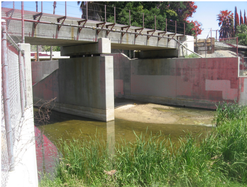
Photograph 20: Arroyo Simi Bridge looking northeast (4/21/2020).
