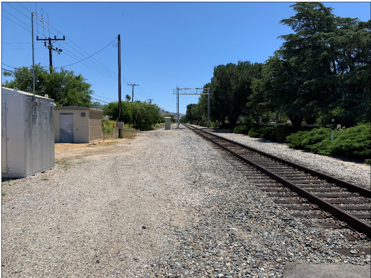
Figure 2-1. Overview of the Southern California Regional Rail Authority Right-of-Way near the Western Extent of the Project Study Area (Facing East)
