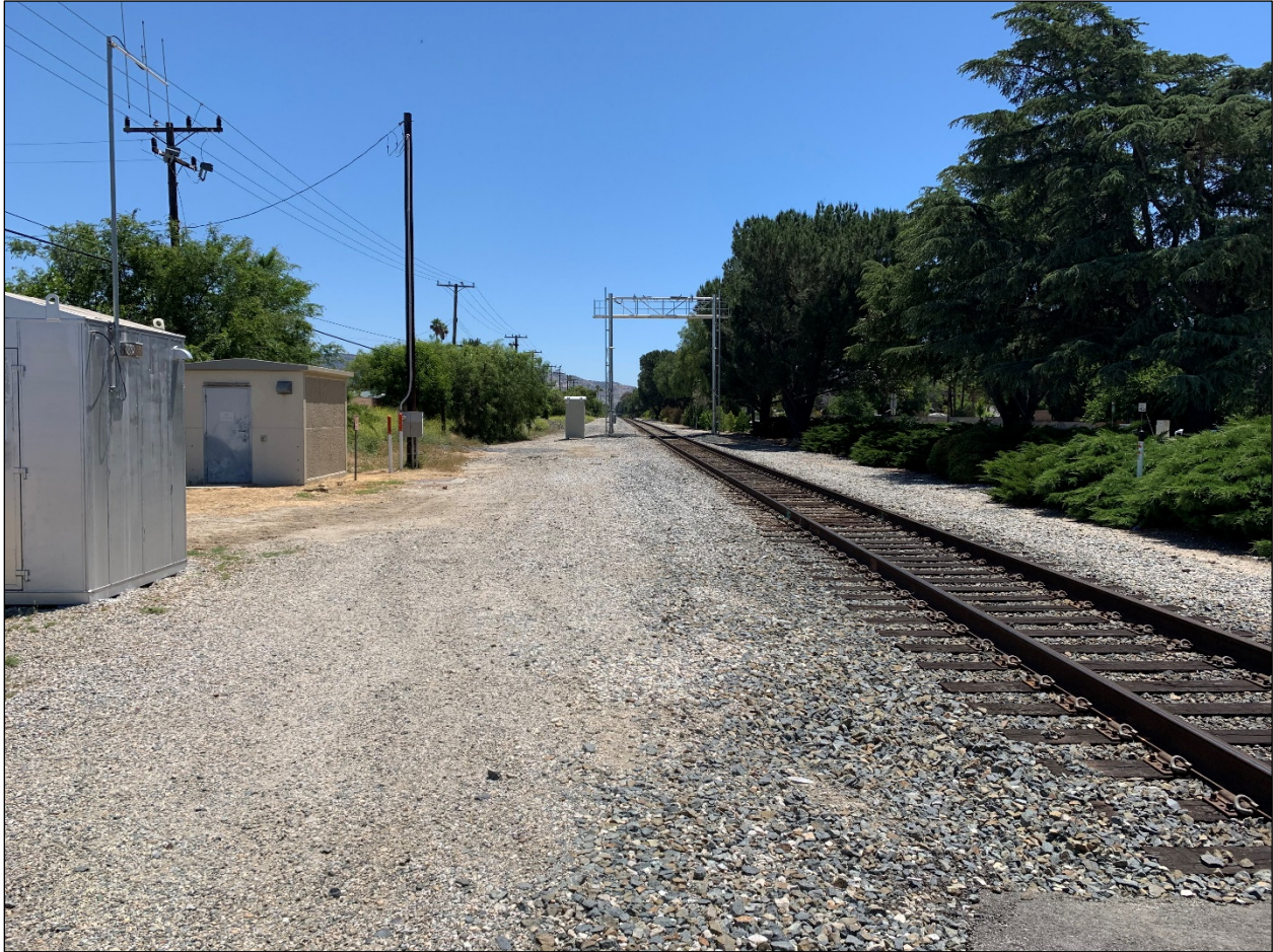
Figure 5-3. Rail Corridor at Topo Canyon Road, Facing East
