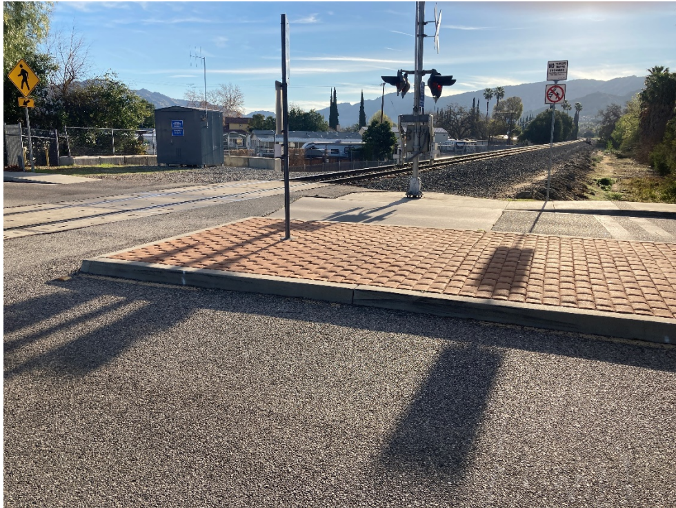
Photo 3: The Hidden Ranch Drive grade crossing had signals and a signal house. The view is to the east.
