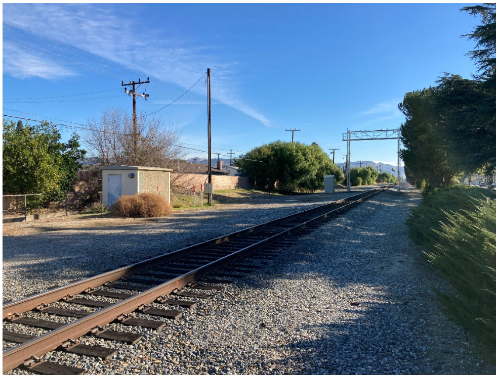
Photo 12: Additional signal and switch houses were located to the east of the Sequoia Avenue grade crossing. Markers for underground fiber optic lines were present throughout the Project footprint. The view is to the east.
