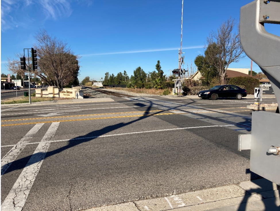
Photo 9: Gates and signals were located at the Tapo Street grade crossing. The view is to the west.
