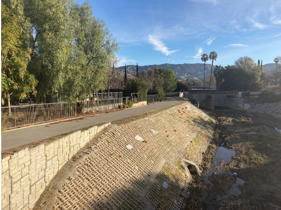
Photo 1: The walking/bicycle path at the eastern extent of the Project footprint was adjacent to a surface drainage channel. The view is to the northeast.
