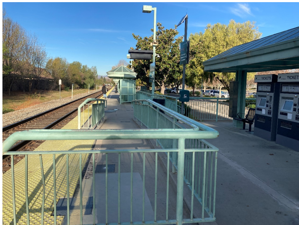
Photo 4: The passenger platform of the Simi Valley Metrolink Station had open canopy structures but no enclosed buildings. The view is to the northwest.
