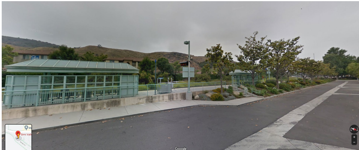
Figure 3.1-2. Key Observation Point 1: Existing Simi Valley Station (Looking West)
